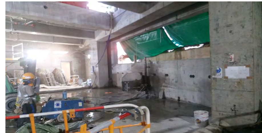
Portion 1 – Saw cut for basement wall at Xiqu Centre
