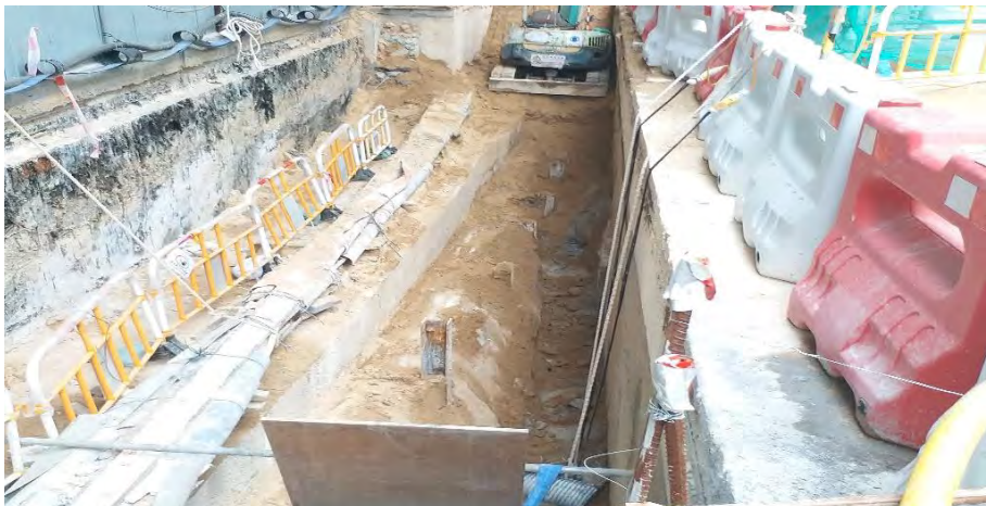
Portion 5 – Excavation for temporary support for DN 900 Drain
