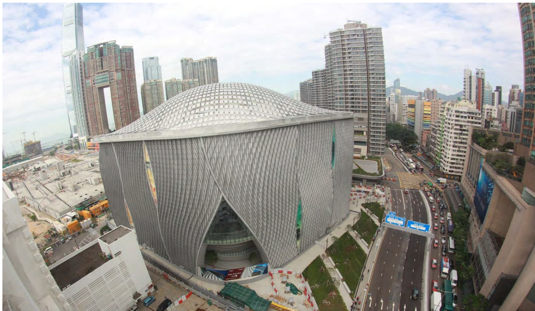
Exterior of Xiqu Centre
