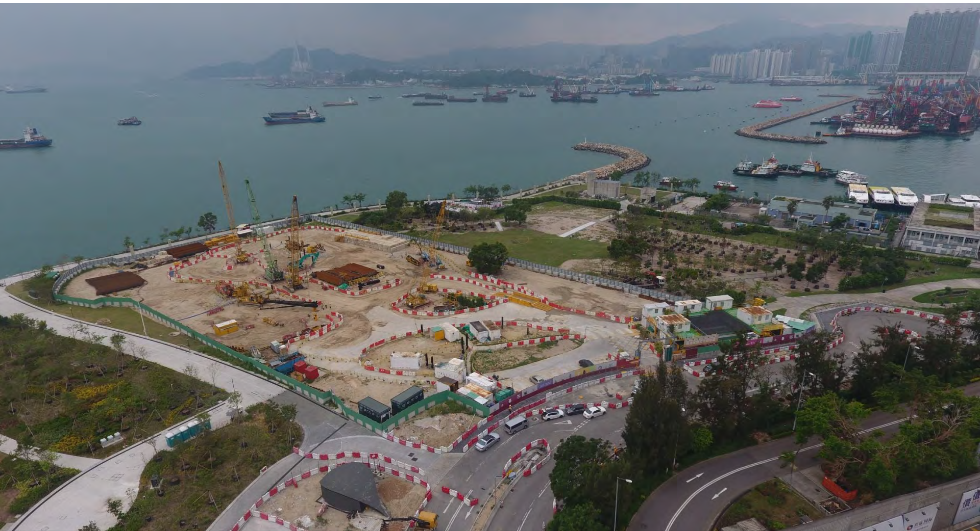
General view for Hong Kong Palace Museum
