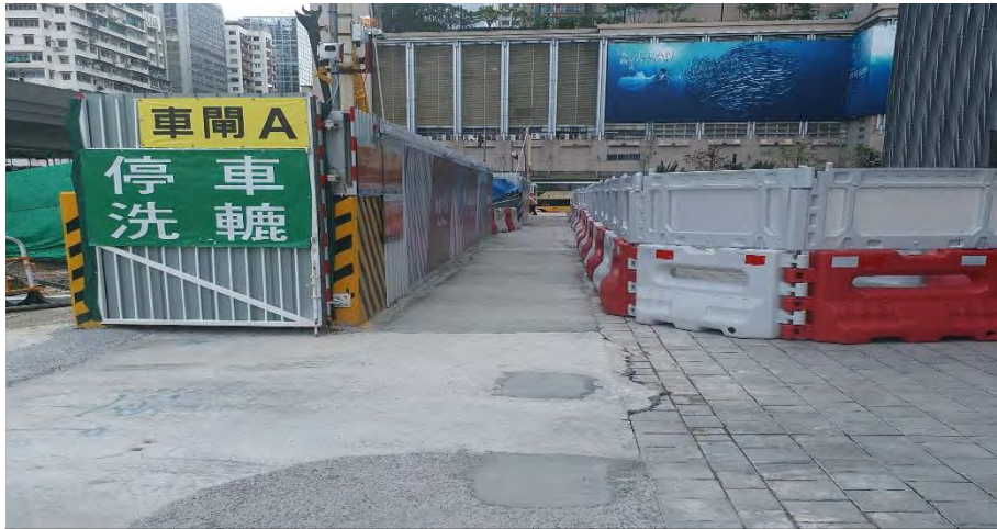
Hoarding at Road Level (Portion 5)
