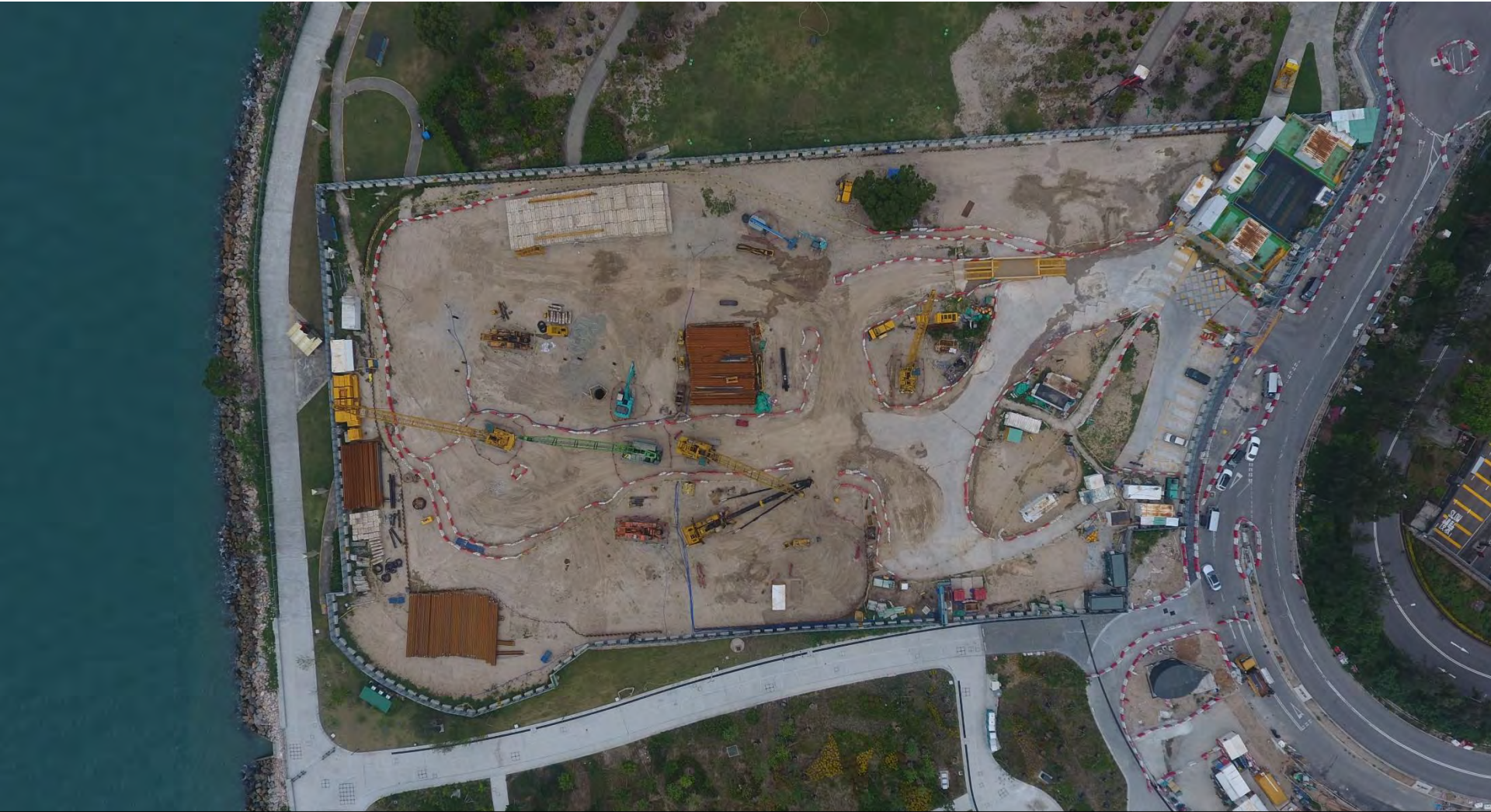
General view for Hong Kong Palace Museum
