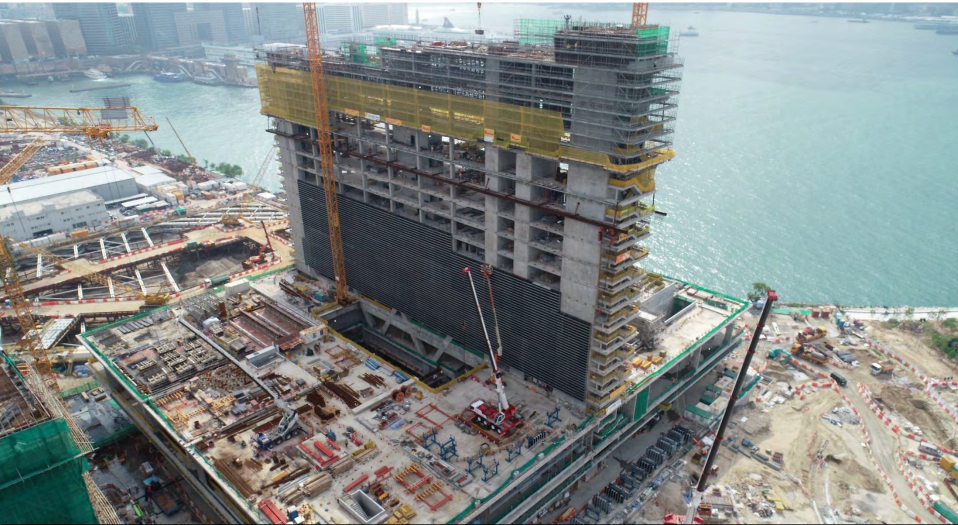
General view of the M+ Tower – Façade (North)
