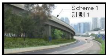
Scheme 1 計劃 1 Proposed single lane elevated road connecting Hoi Po Road to West Kowloon Highway northbound 擬建高架單線行車道連接海寶路至西九龍公路北行方向
