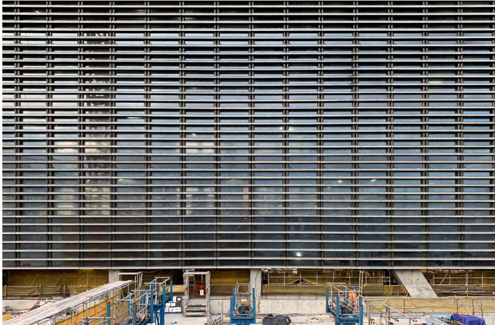
M+ Tower – Façade View from 3/F M+ 縱向大樓 — 3樓外牆概覽
