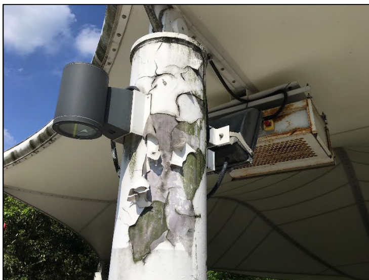
Column with paint peeled off at amphitheatre
