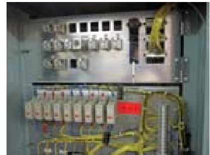
Obstruction Switch installed in the Control Panel
