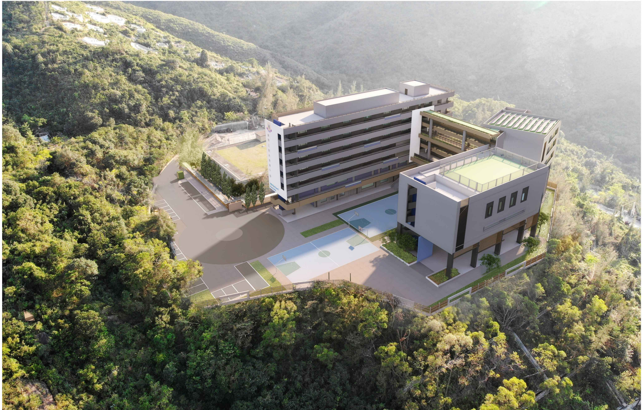
從東北面望向小學的構思圖 VIEW OF THE PRIMARY SCHOOL FROM NORTHEAST DIRECTION
