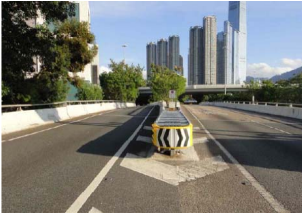
Installing crash cushion
