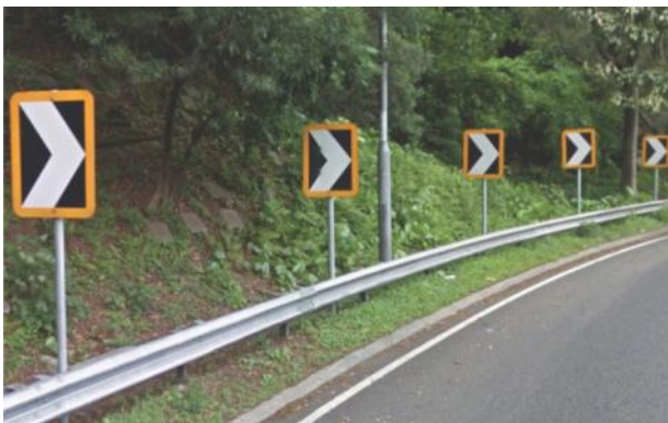
Installing warning traffic signs at road section with sharp bend
