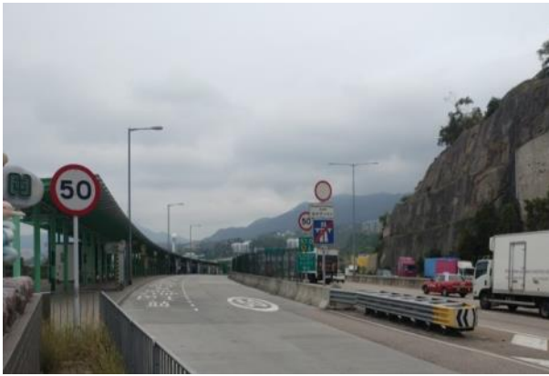
Installing safety barrier at bus interchange to separate main carriageway
