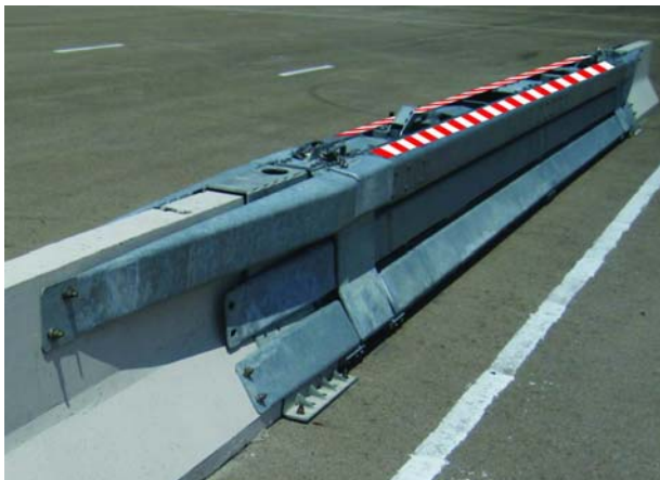
Installing movable safety barrier at emergency opening at central medium
