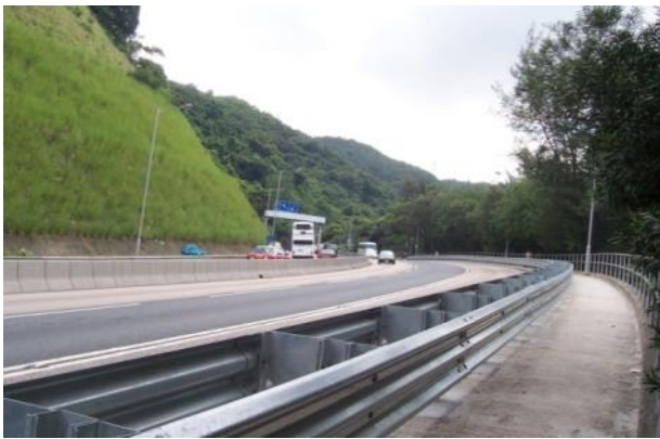
Reinforcing safety barrier
