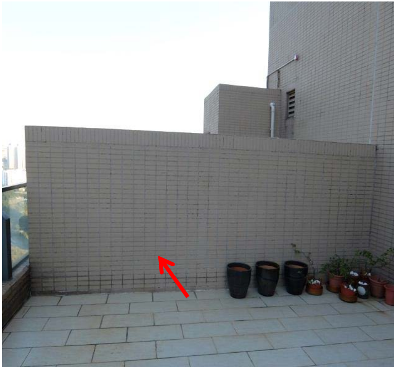
實心牆 (建築物屋頂) Solid fence wall (on roof)
