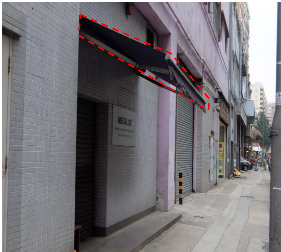
可收合的遮篷 (平台/天台上或街道上) Retractable awning (over a roof or a street)
