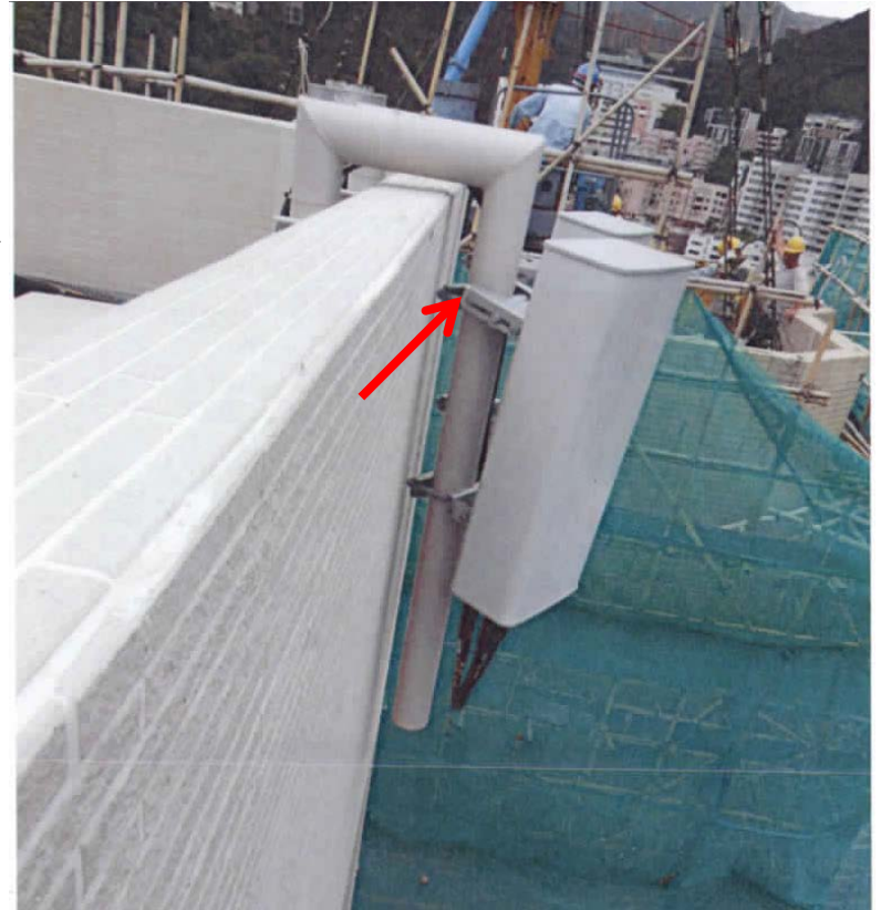
(外牆) (External Wall)
