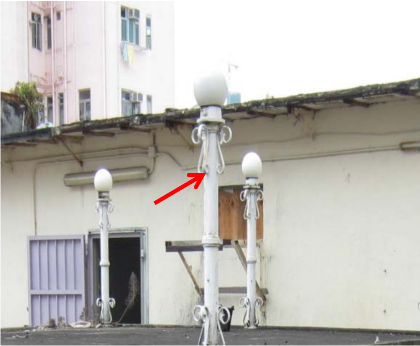
支柱 (建築物屋頂) Pole (on roof)
