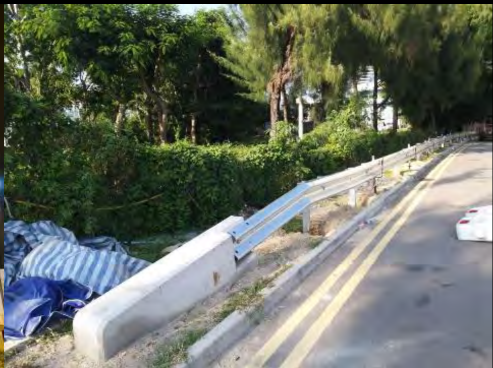
Installation of Untensioned Beam Barriers
