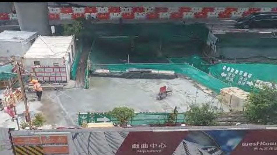
Backfilling works for MOE staircase 逃生梯的回填工程
