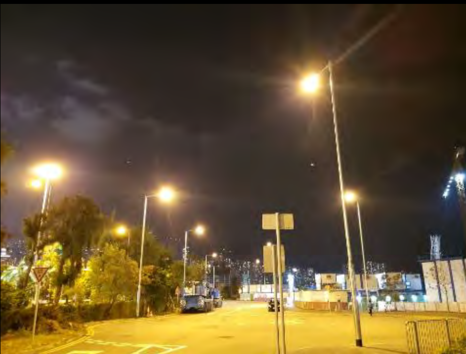
Completion of Road Lighting at U-shaped Haul Road
