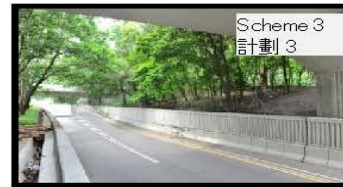
Scheme 3 計劃 3 Proposed single lane at-grade road connecting West Kowloon Highway southbound to elevated Nga Cheung Road 擬建地面單線行車道連接西九龍公路南行方向至雅翔道高架路段
