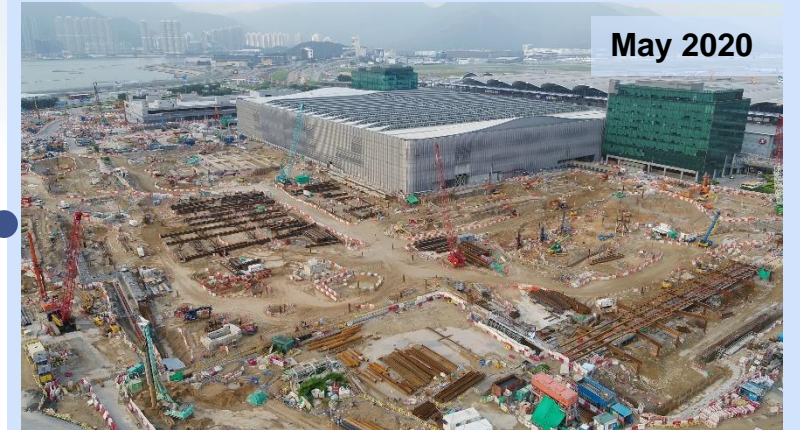
T2 Expansion Advance Works
