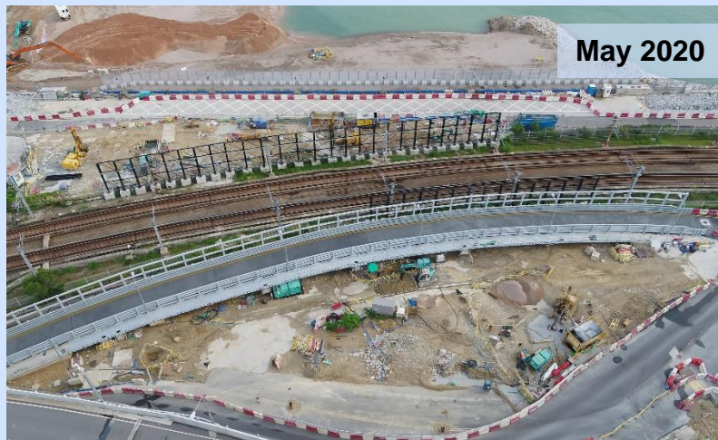
Tunnel works under AEL
