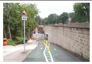
Additional safety facilities at sharp bends to alert the cyclists to slow down and segregate two-way cycling traffic
