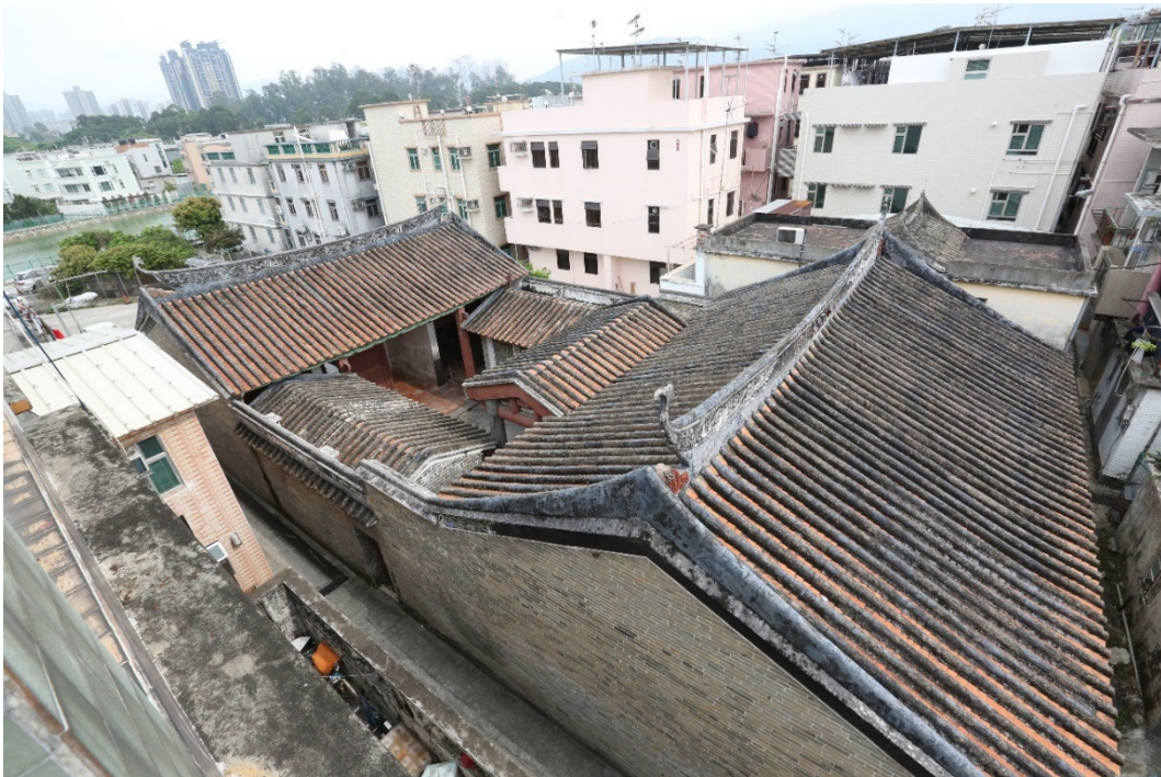
Two-hall-three-bay layout with the rear hall fronted by a porch with humpbacked roof
