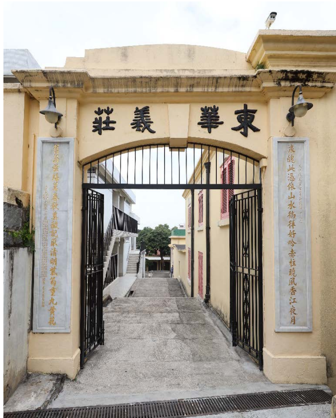
A Western-style segmental pai fong (牌坊) at the coffin home. The structure is topped by a cornice with a slightly curved pediment above. The name “Tung Wah Coffin Home” is moulded in relief in Chinese to either side of the keystone.
