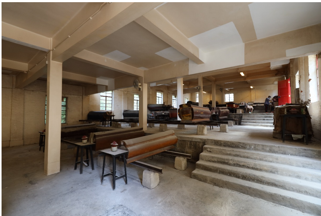
Interior of the New Hall. It is a flat concrete roofed building supported by rectangular columns.
