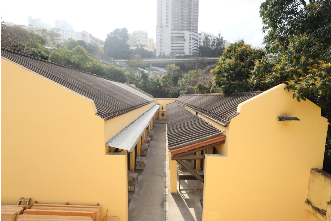
The coffin rooms “Hong” (left) and “Ning” (right) were built with pitched roofs laid with double pan and roll tiles.
