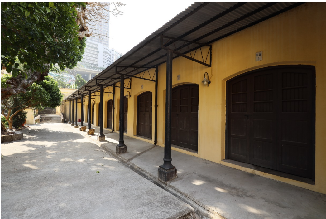
The verandah in front of the “Sau” coffin room supported by iron columns and brackets
