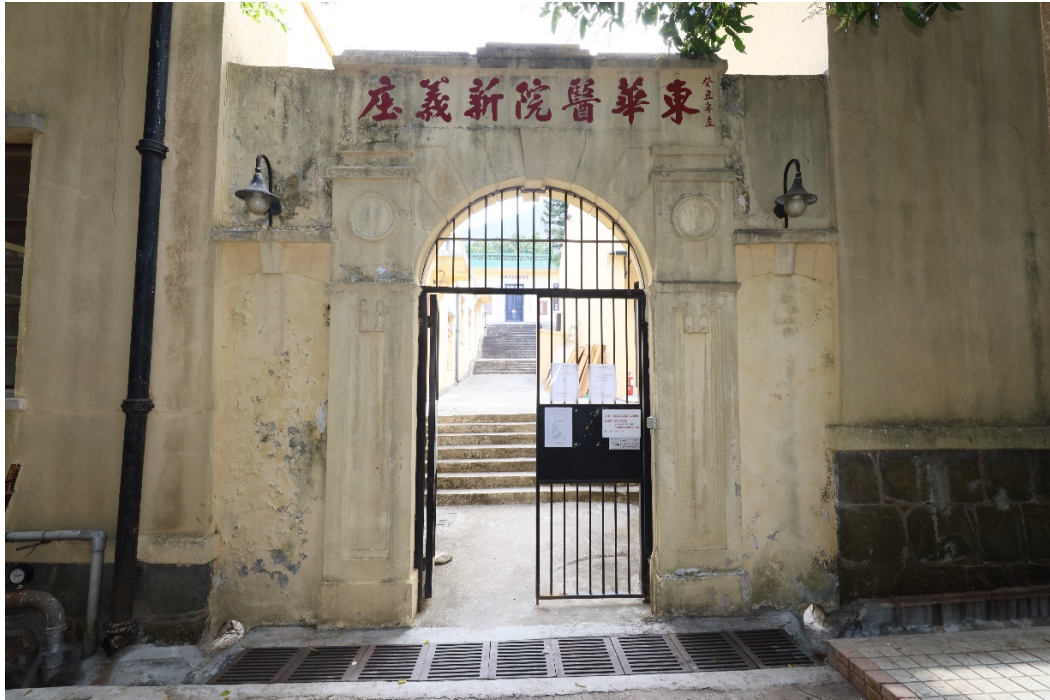
The western entrance of the coffin home built in 1913. The central bay is decorated with moulded voussoirs, a keystone and a pair of ornamental pilasters.
