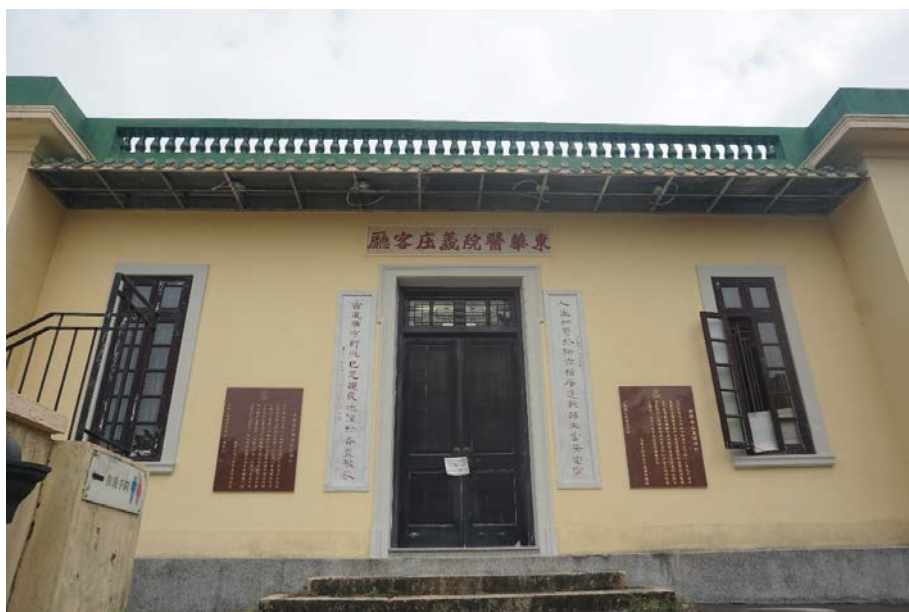
Front elevation of the Reception Hall. The parapet on the concrete flat roof is decorated with vase-shaped balusters.
