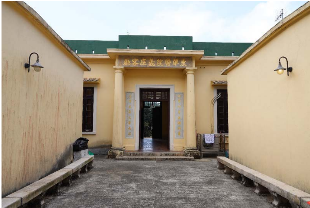
Rear elevation of the Reception Hall. A portico is supported by a pair of Tuscan columns and pilasters.
