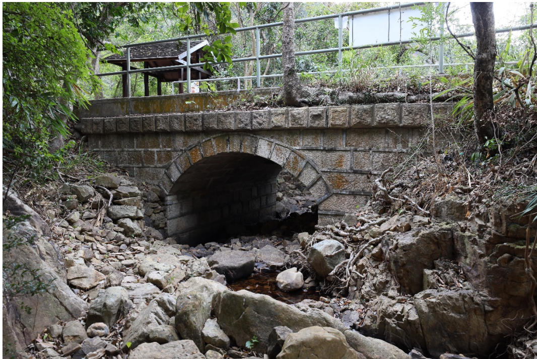
North elevation of the Masonry Bridge
