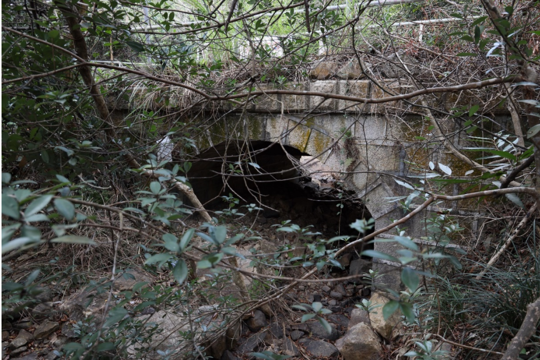
South elevation of the Masonry Bridge
