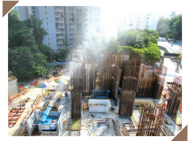
A mist jet gun helps lower the temperature on a site
