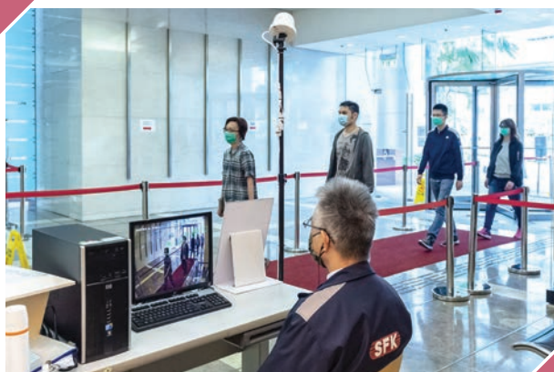
Temperature scanning systems have been installed at entrances to the HAHQ
