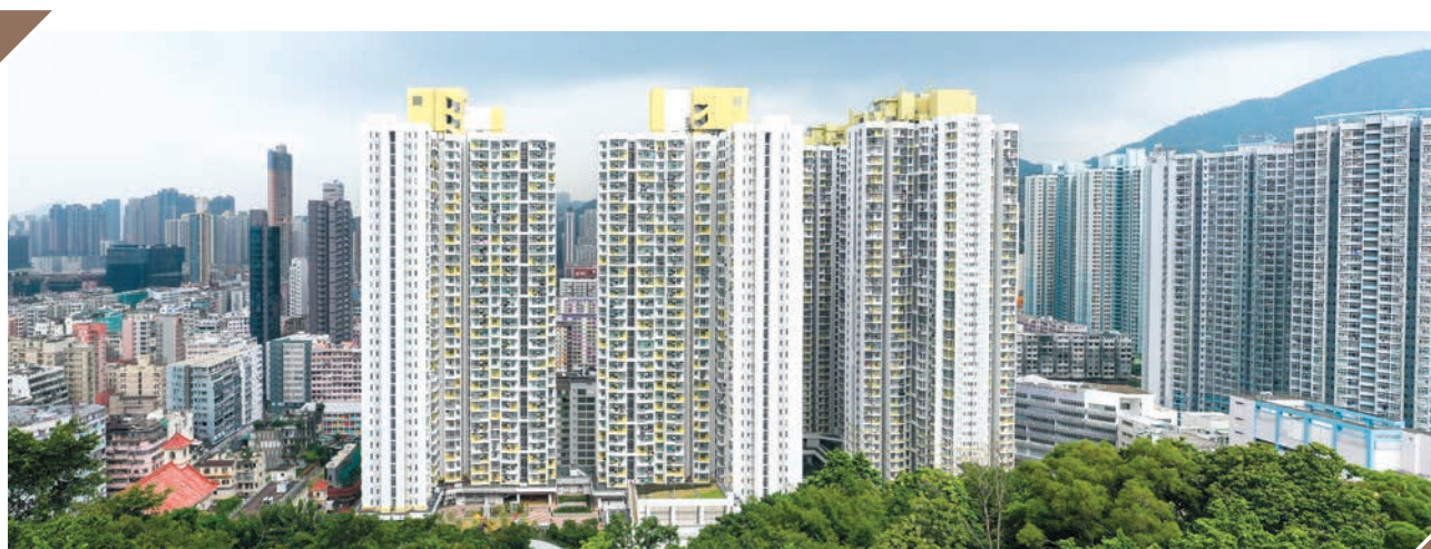
Shek Kip Mei Phase 6 (two blocks on left)
