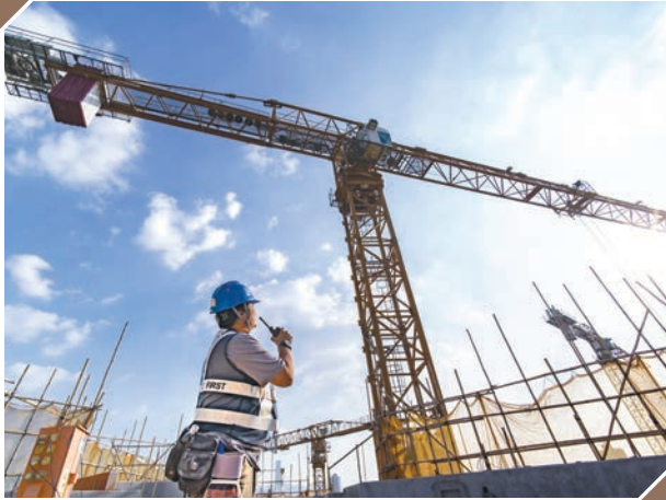
A worker working under the tower crane
