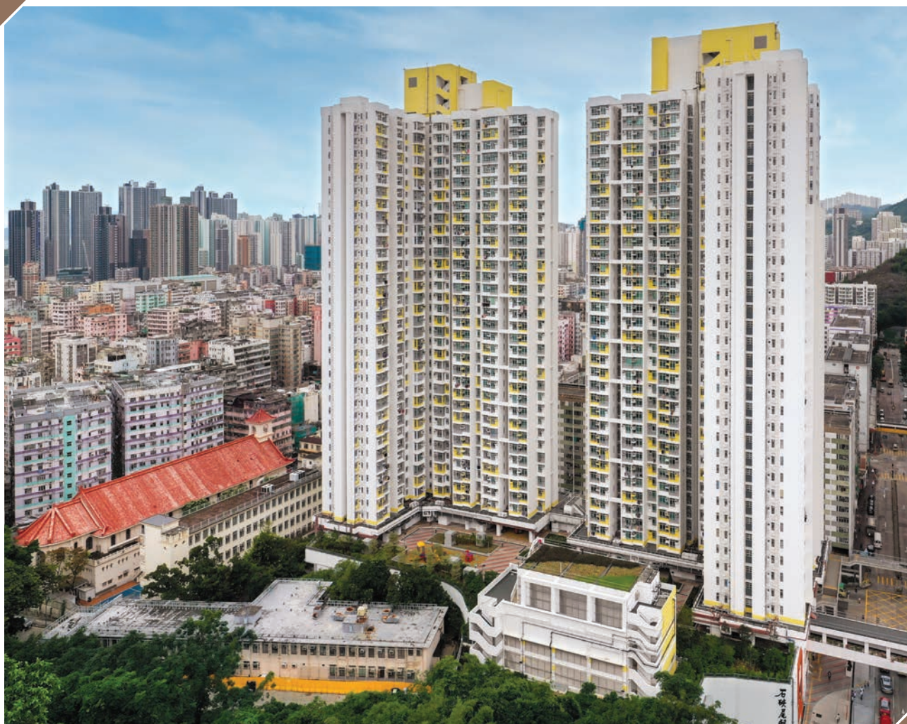
The newly completed PRH project – Shek Kip Mei Phase 6
