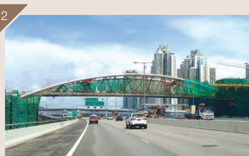
Finishing works on the footbridge (June 2020)
