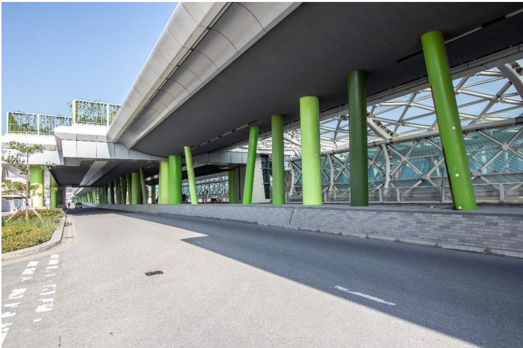
Shing Fung Road
