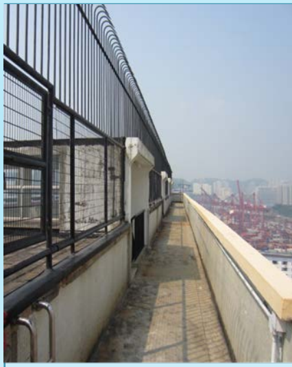
網欄或金屬欄杆 Mesh fence or metal railing
