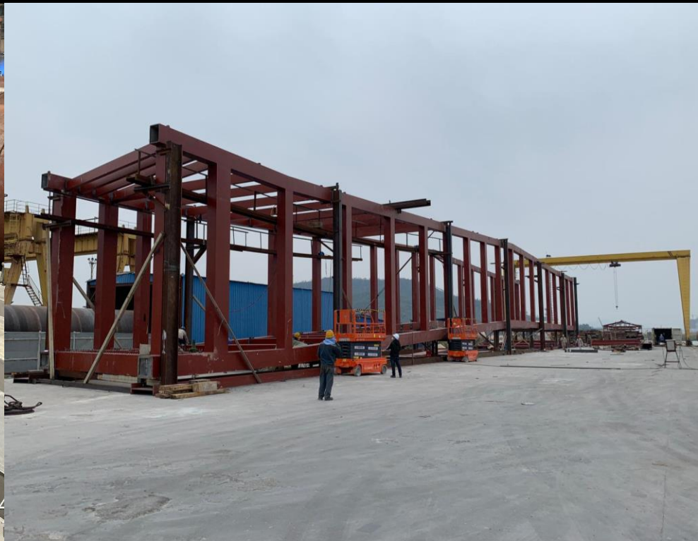
Installation of bottom cross beams 安裝底部橫樑
