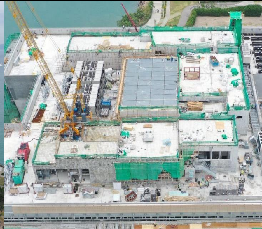
Roof Skylight Installation Works Completed 天台的天窗安裝工程完成
