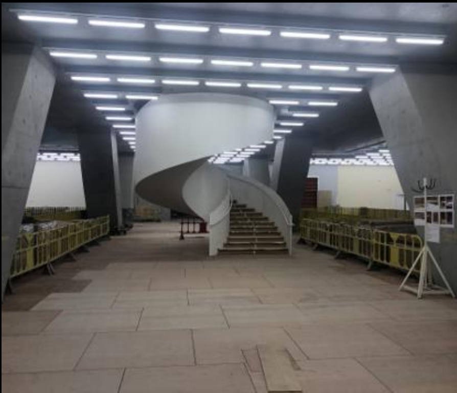
2/F Atrium Timber Progress 2 樓中庭鋪設木地板進展
