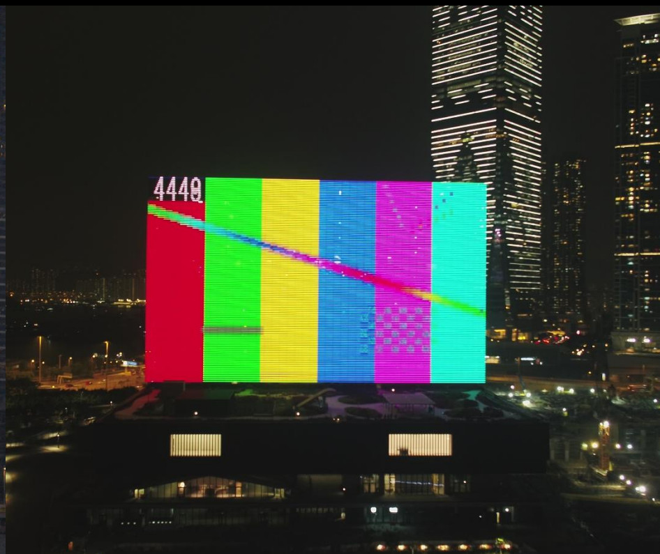
M+ LED Façade Lighting Testing M+ LED幕牆燈光測試
