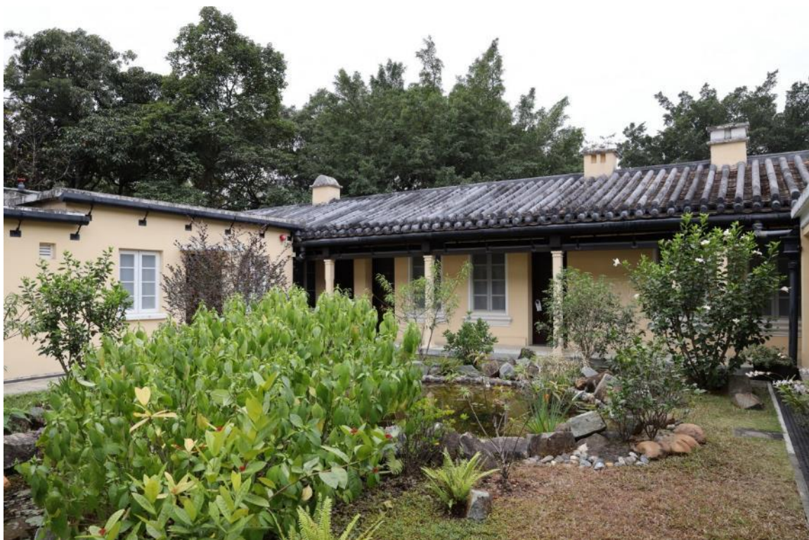
Chinese-style pitched roofs covered with pan and roll tiles at the Main Building, chimneys can be seen on the roofs
