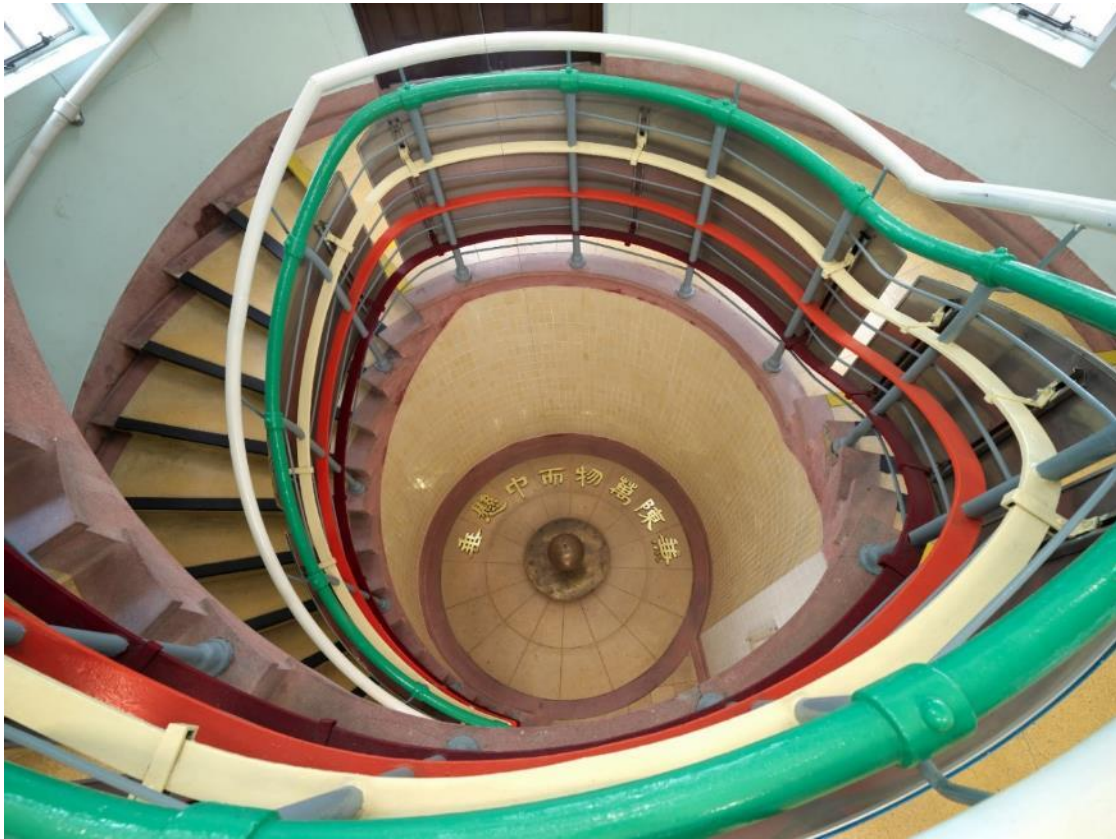
The central spiral staircase with terrazzo finishes
