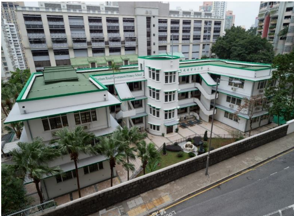
Bird's eye view of the main building of Bonham Road Government Primary School, showing its E-shaped plan comprising a long centre portion and a wing on each end
