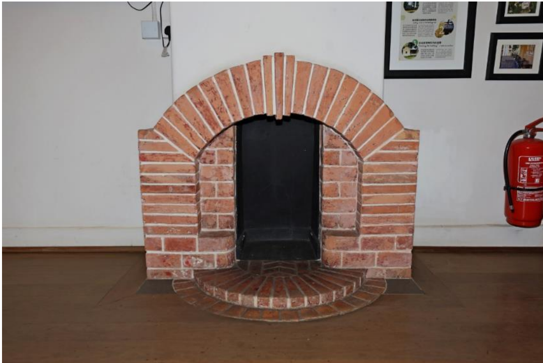
Fireplace at the Main Building
