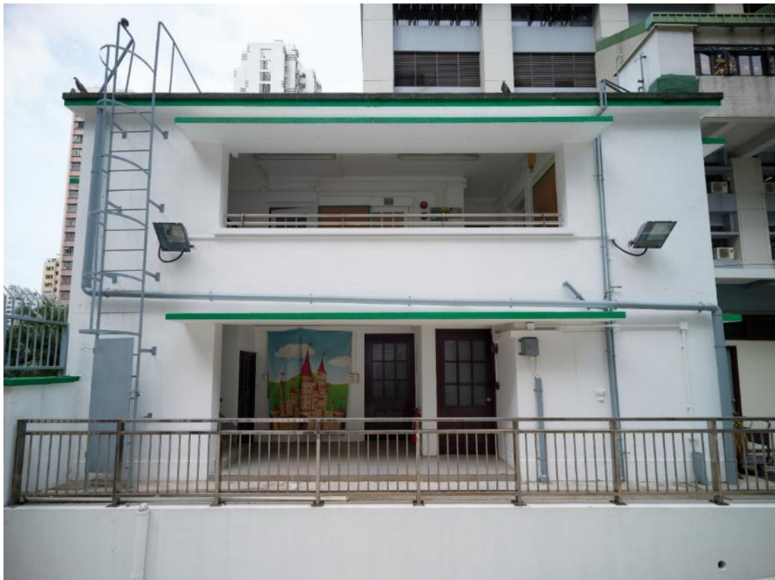
The two-storey former caretaker's quarters situated near the entrance gate on Eastern Street
