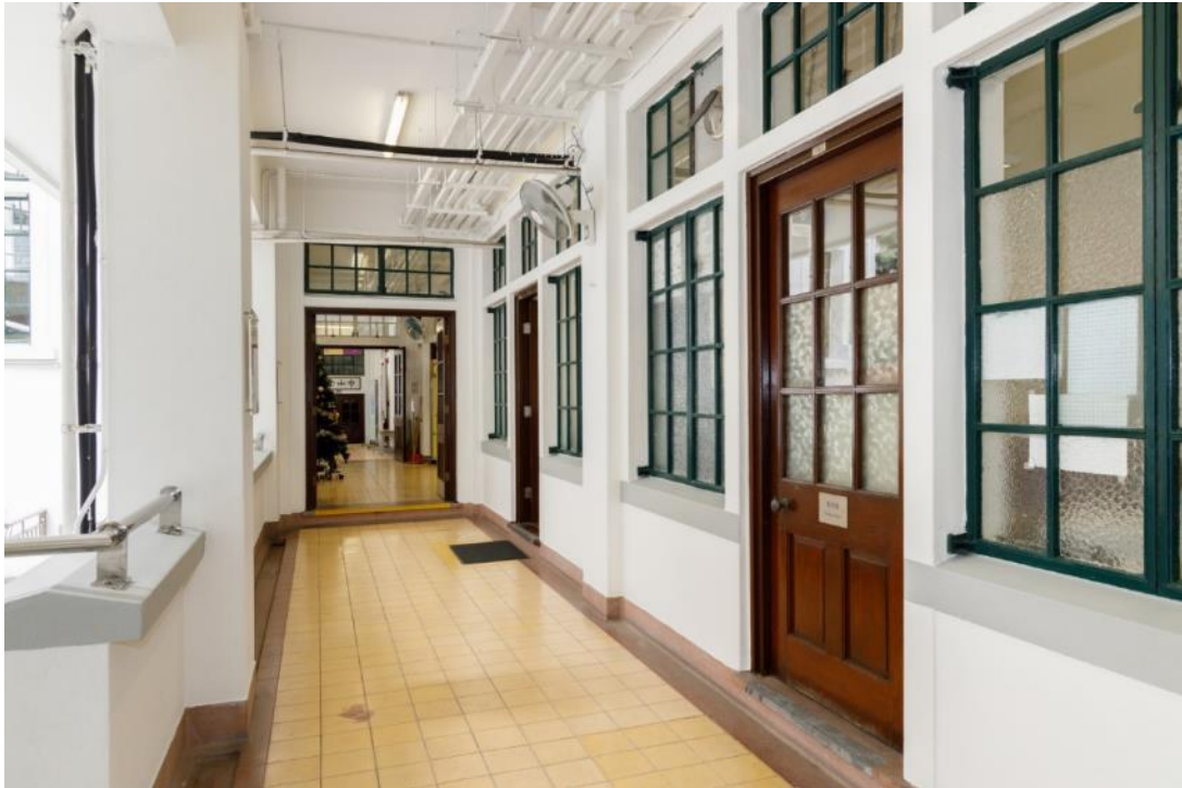
The timber doors, steel-framed windows with patterned or plain glass panes, and the old-styled ironmongery are all well maintained.
