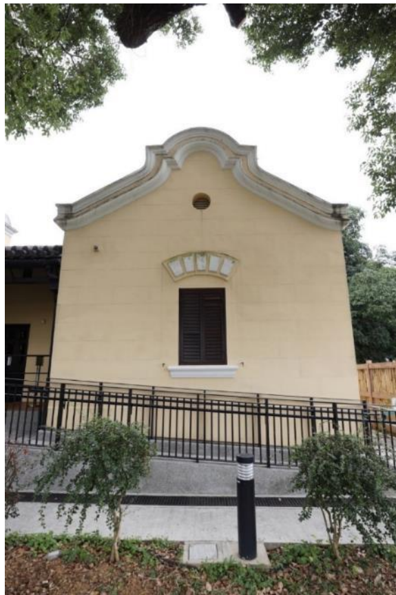
Dutch gables with oculus and five voussoirs above the windows at the Main Building
