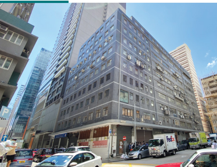
Retrofitting works to be carried out at Yu Chau West Street Project allows the URA to explore retrofitting initiatives to extend the serviceability of old industrial buildings.
