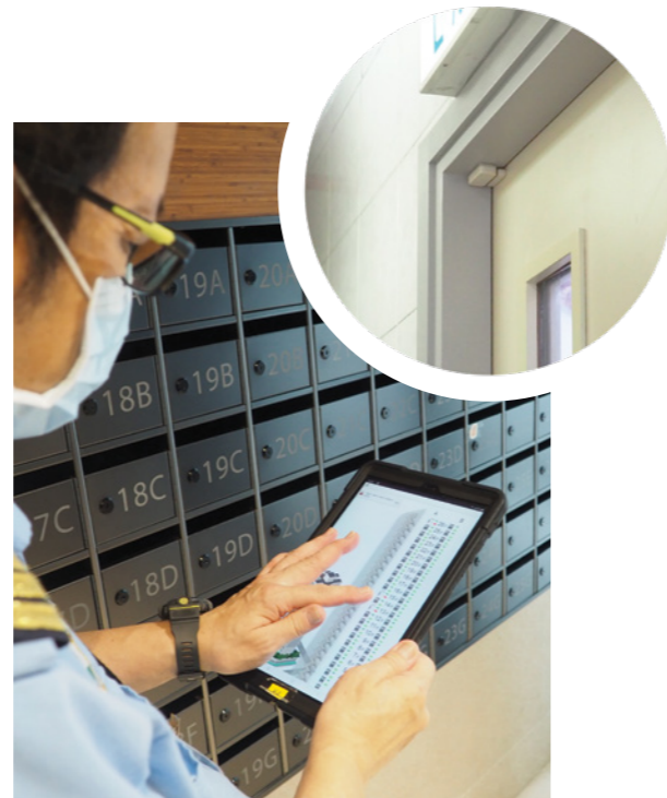
Digital remote monitoring units installed at URA's rehousing block
