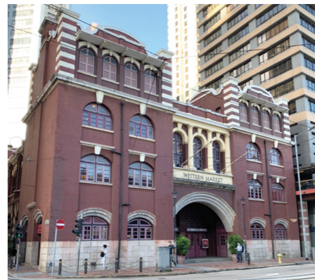
Current view of the Western Market
