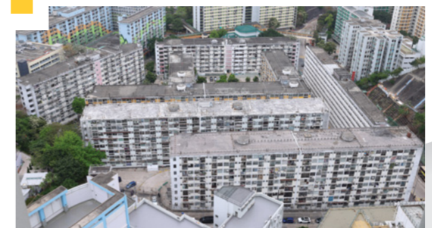
The aerial view of Tai Hang Sai Estate
