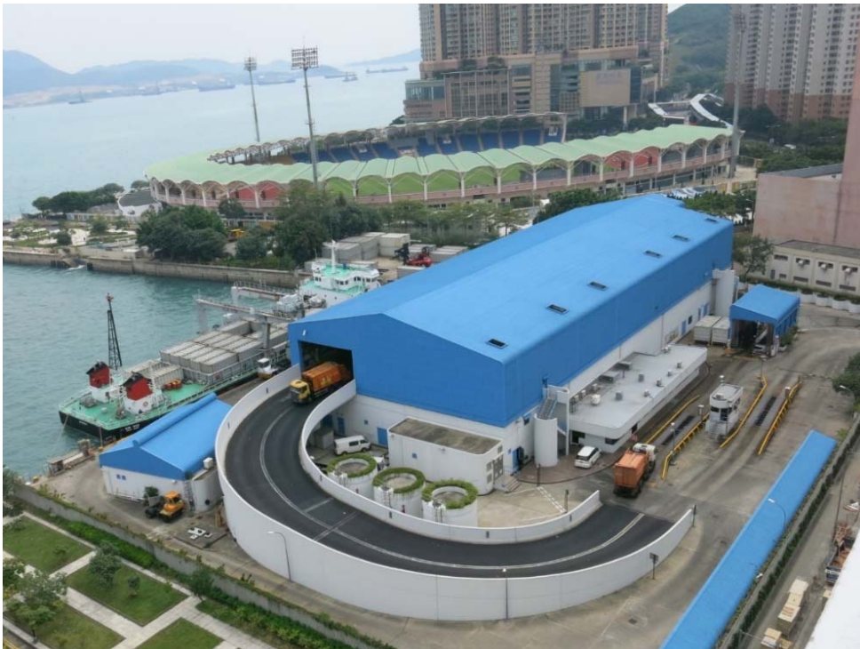
Figure 2 Island East transfer station
