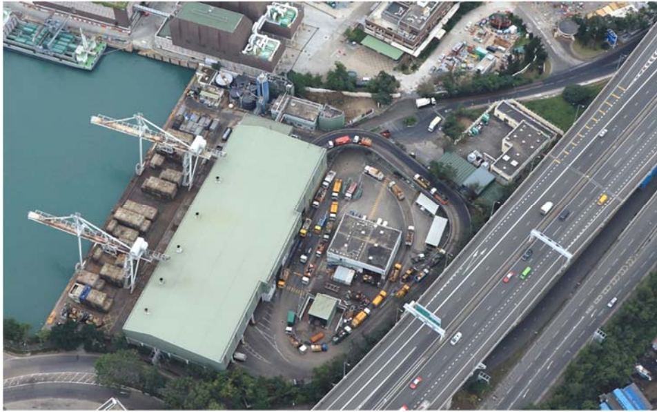
Figure 1 West Kowloon transfer station
