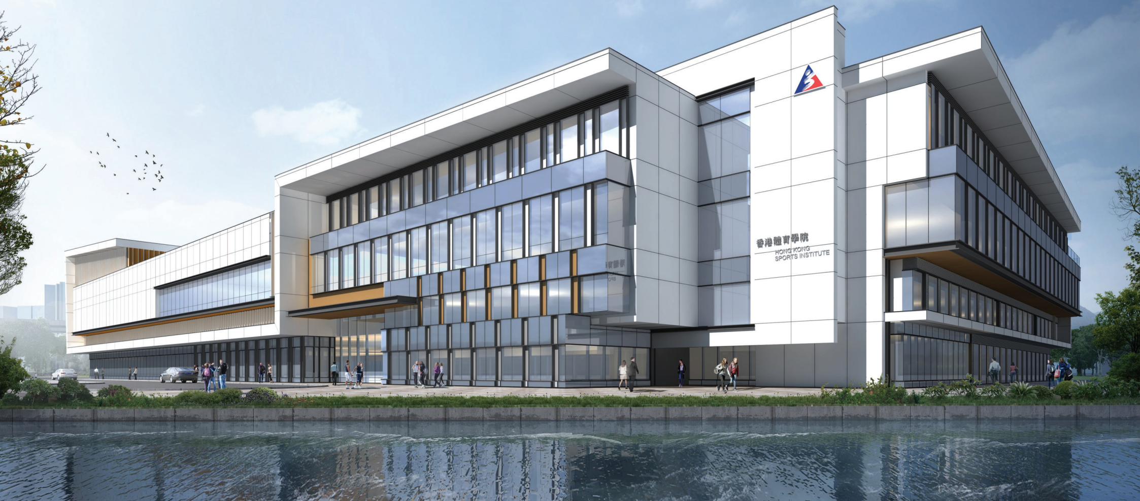
從城門河岸望向大樓的構思圖 PERSPECTIVE VIEW FROM SHING MUN RIVERBANK (ARTIST'S IMPRESSION)
