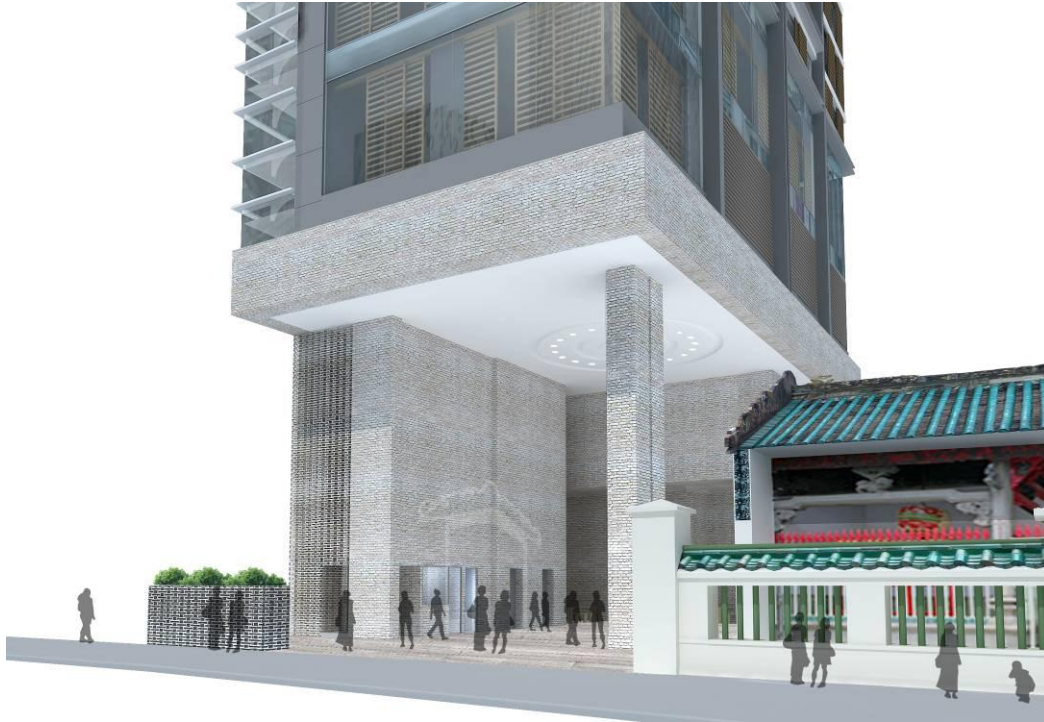
Figure 7: Perspective showing the further setback of the stair core at ground floor by approximately 5 800 mm.
