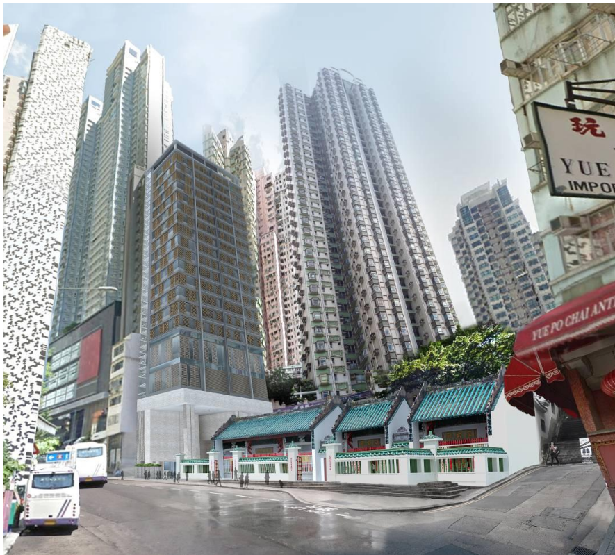
Figure 5: The entire building is set back from Hollywood Road.
