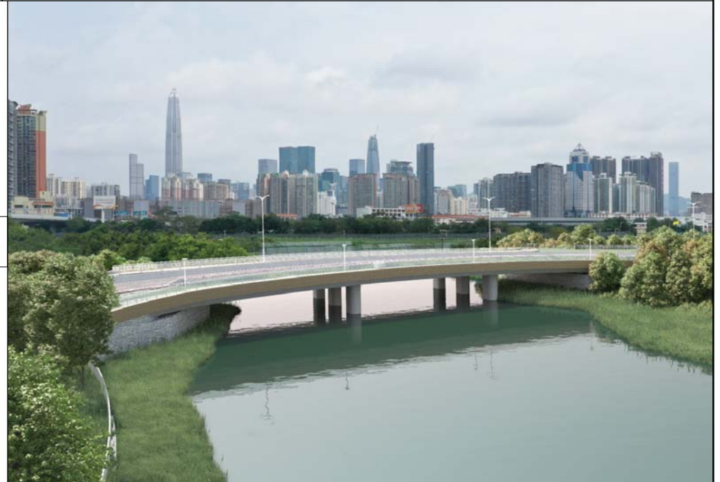
擬議跨越河曲行車橋 (包括雙程雙線分隔道路、行人路及單車徑) PROPOSED MEANDER BRIDGE (INCLUDING A DUAL TWO-LANE CARRIAGEWAY, FOOTPATH AND CYCLE TRACK)
