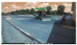
LSCM and a local university have jointly developed a technology using computer vision and machine learning to automate the existing quality management process which relies heavily on manual operation and records. The technology will analyse images of site activities captured real-time by surveillance cameras and utilise machine intelligence to determine if there are any quality deviations and/or defects.
