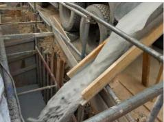
NAMI has developed a self-leveling, free-flowing, soil-like backfill material. Unlike conventional soil-based backfilling requiring layer-by-layer soil compaction, the flowable fill material can continuously be pumped into the trench, enhancing productivity and pavement quality.
