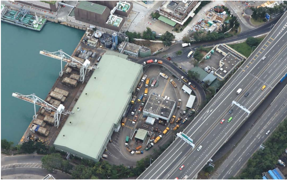
Figure 1 West Kowloon Transfer Station
