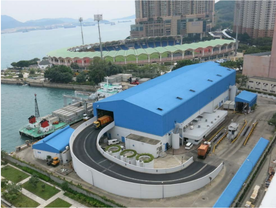
Figure 3 Island East Transfer Station
