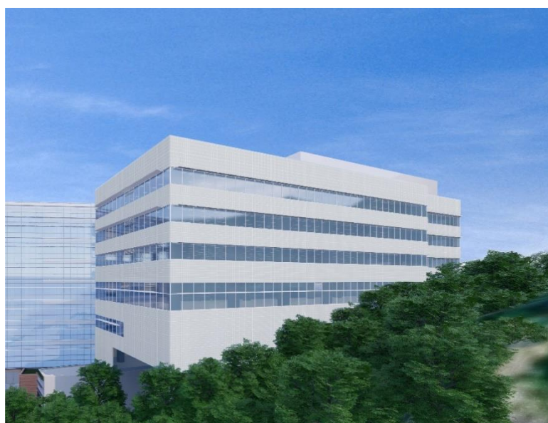
從西南面望向大樓的構思圖 View of the building from southwest (Artist's impression)
