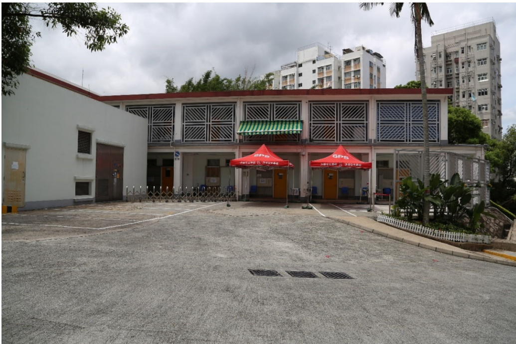
Figure 4: Existing parking spaces in school
