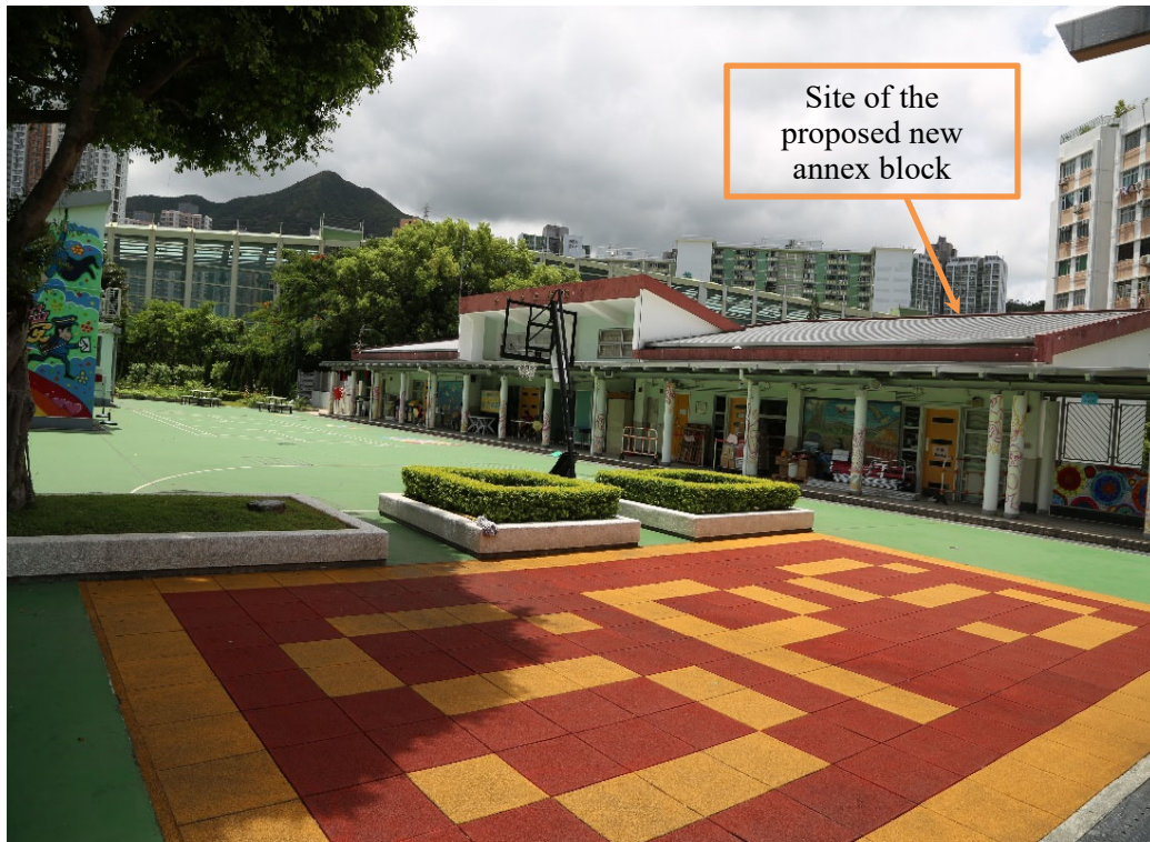
Figure 5: Existing basketball court and the one-storey school building (mainly staff room and activity room)
