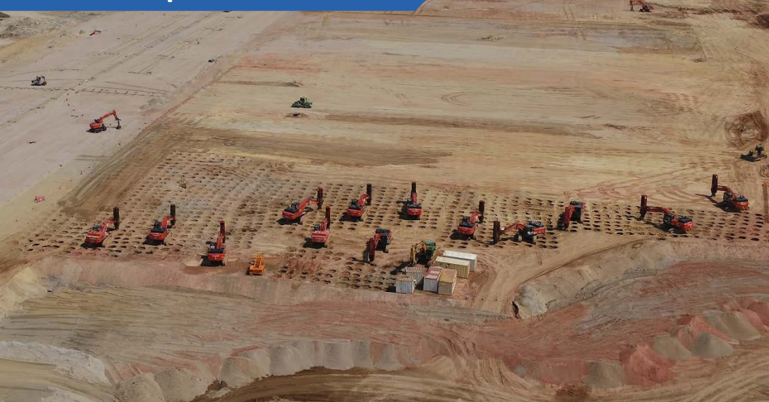
Ground Improvement works
