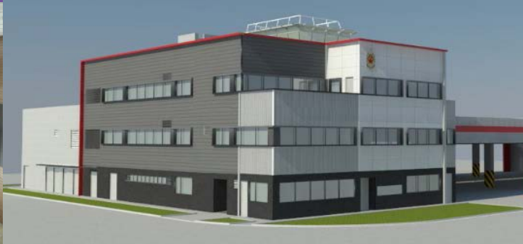
New West Fire Station
