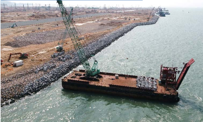
Laying of Accropode
