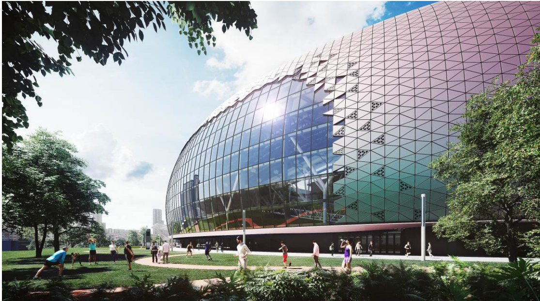
Figure 4: Gigantic glass wall at Main Stadium south stand
