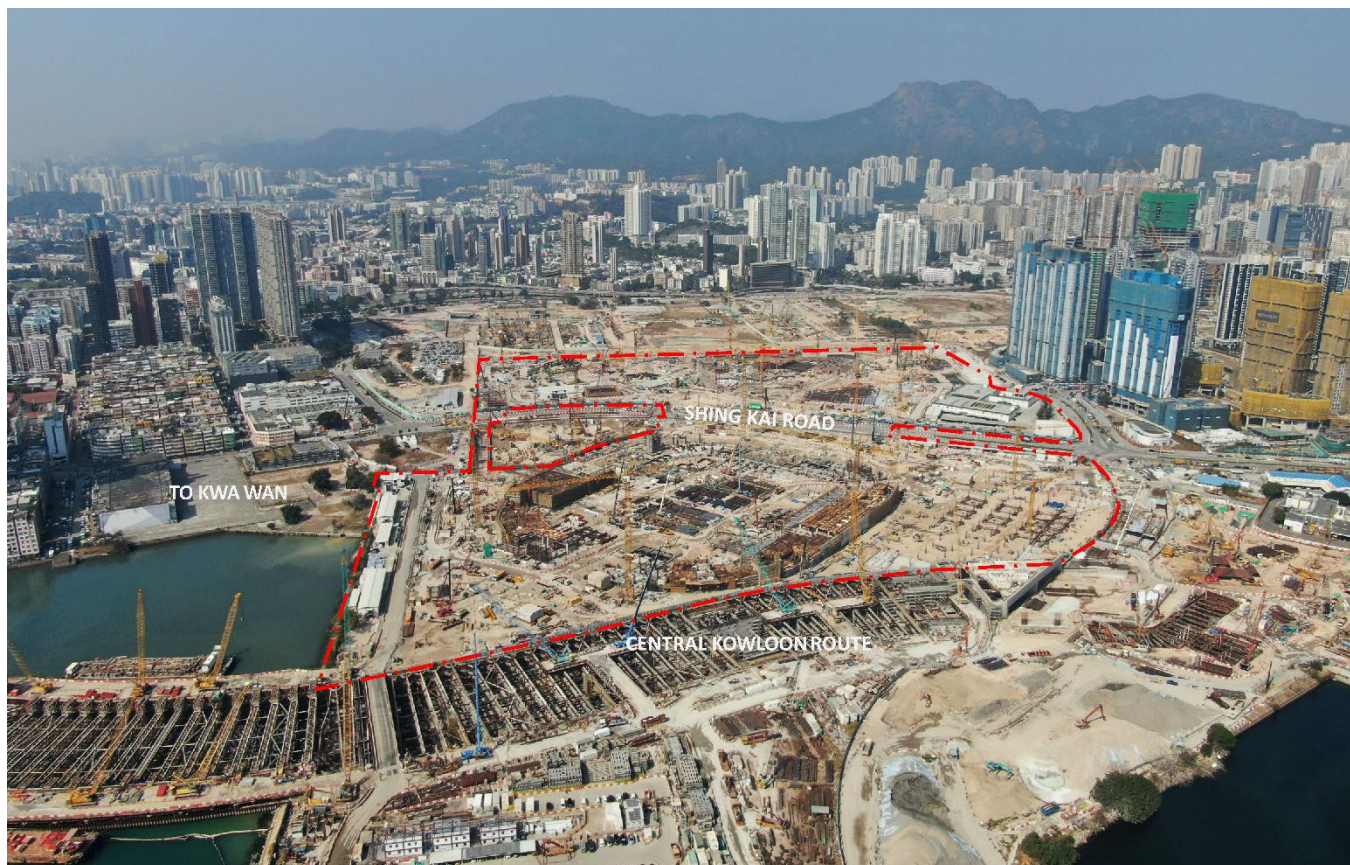
Figure 9: Construction Progress Photo
