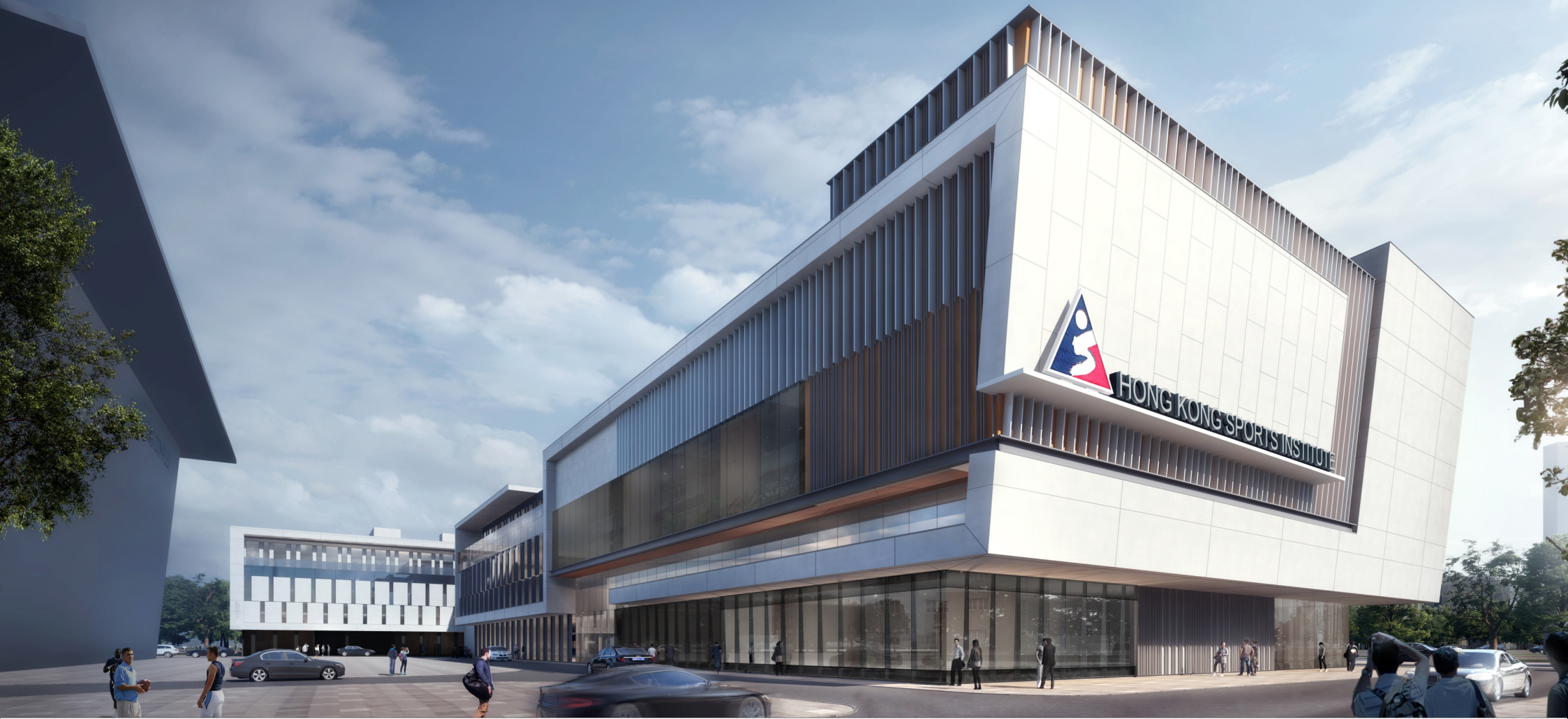
從主大樓望向大樓的構思圖 PERSPECTIVE VIEW FROM MAIN BUILDING (ARTIST'S IMPRESSION)
