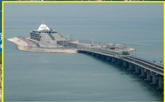
海底隧道及人工島 Subsea Tunnel and Artificial Island
