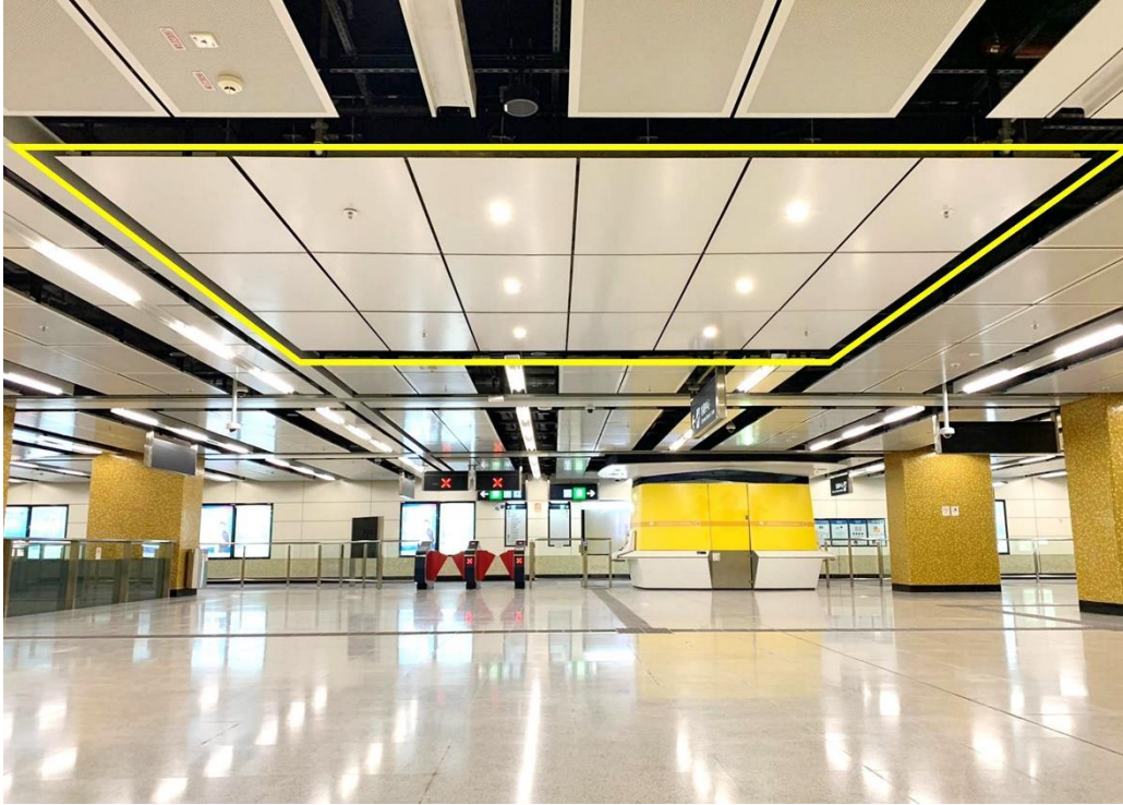
Location of the concrete well trough covered by station ceiling panels
