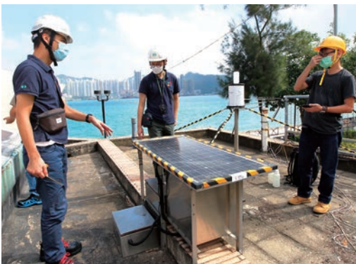
職安局的專業顧問團隊正就天文台設置和更換光伏板的工序作風險評估。 Our professional consultant team performed risk assessment of the setting up and replacement of the photo-voltaic panel at an experimental automatic weather station.
