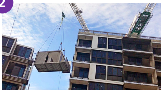
採用「組裝合建築」方法，減低碳排放 Use MiC method to reduce carbon emissions
