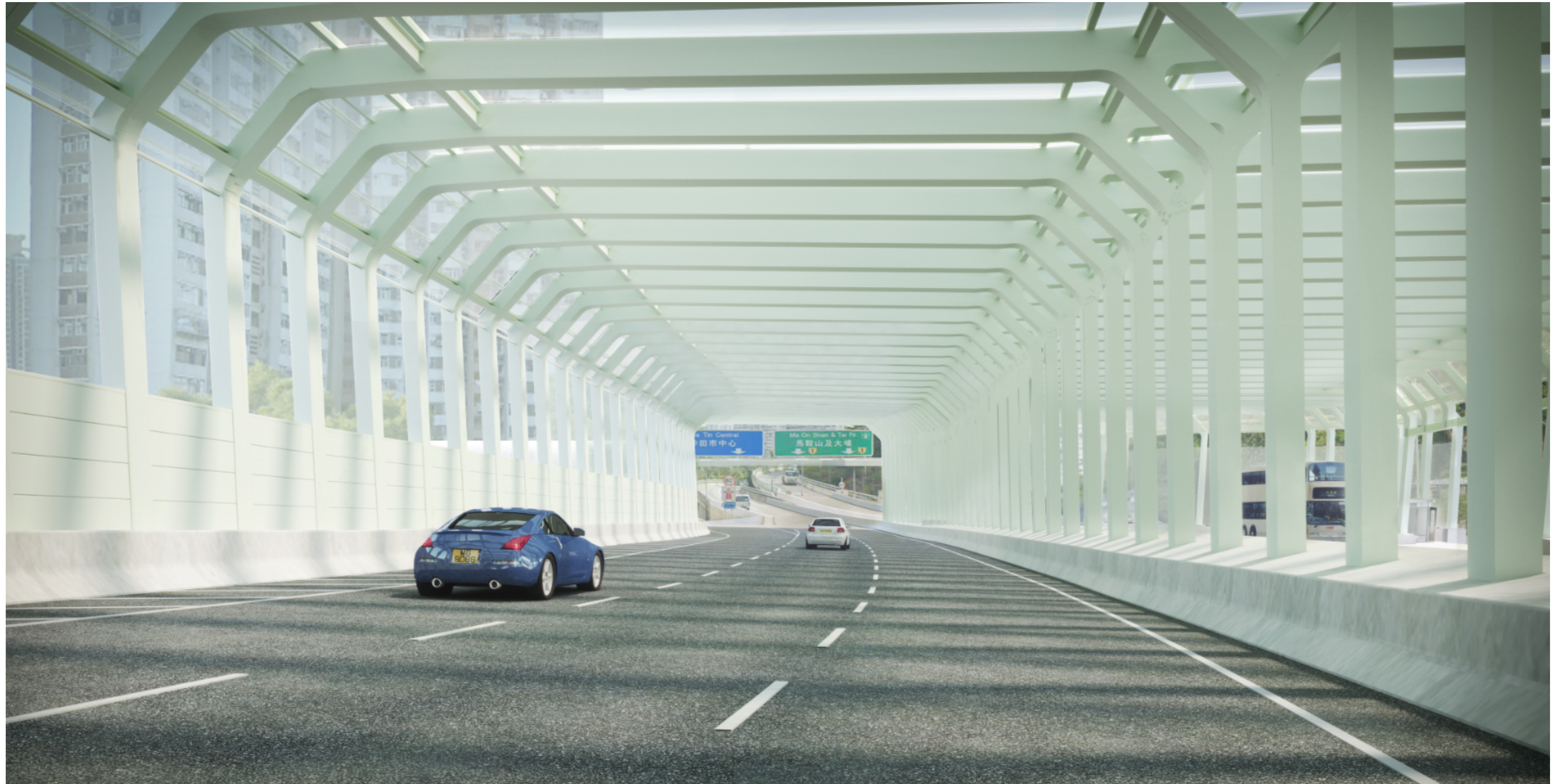
近豐盛苑擬議隔音罩內觀圖 INTERNAL VIEW OF PROPOSED NOISE ENCLOSURE NEAR FUNG SHING COURT
