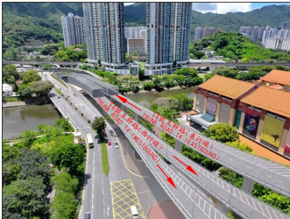
橫跨城門河道的高架行車道 Elevated Carriageway Across Shing Mun River Channel
