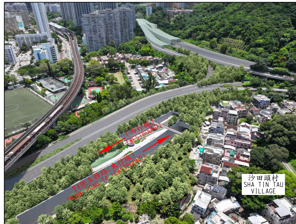
近沙田頭村的地下行車道 Underpass near Sha Tin Tau Village
