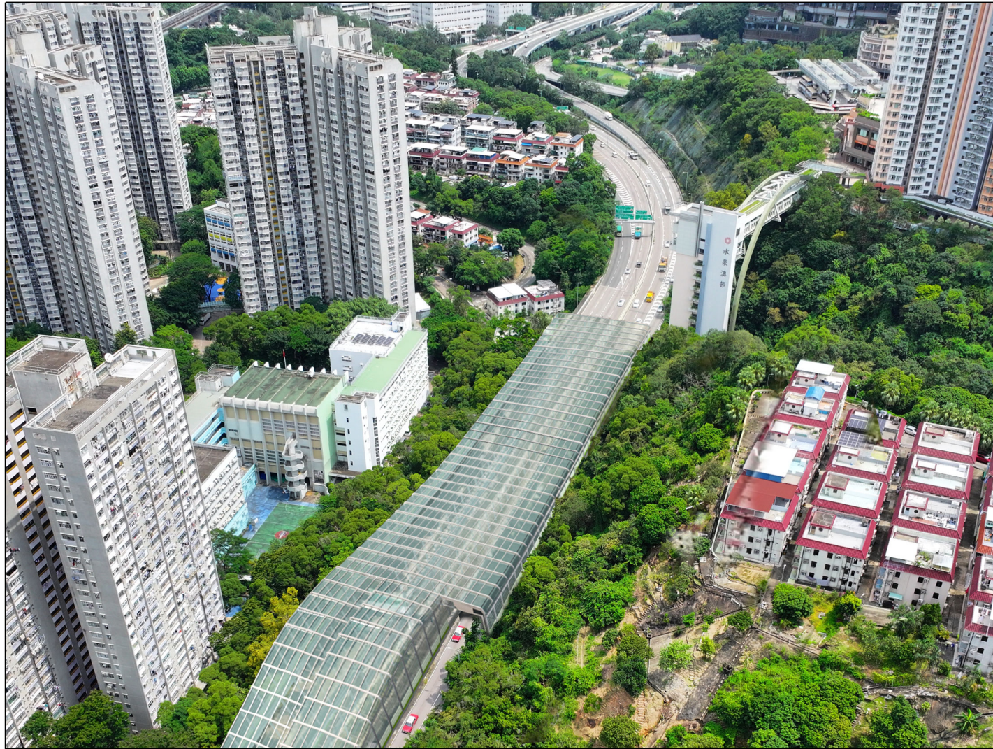
位於沙田路的擬建密封式隔音屏障 Proposed Full-Enclosure Noise Barrier at Sha Tin Road
