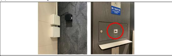
A user counting device and a sanitary fitment occupancy sensing device (as highlighted)
