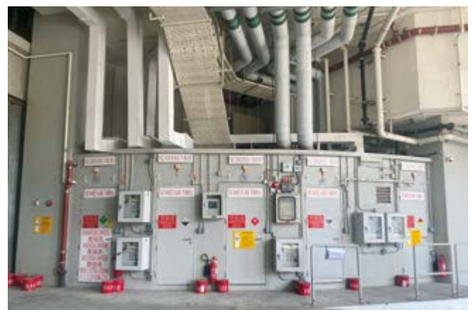
The new Dangerous Goods Store in the Theatre Block. 新危險倉庫設於劇院大樓地下高層。
