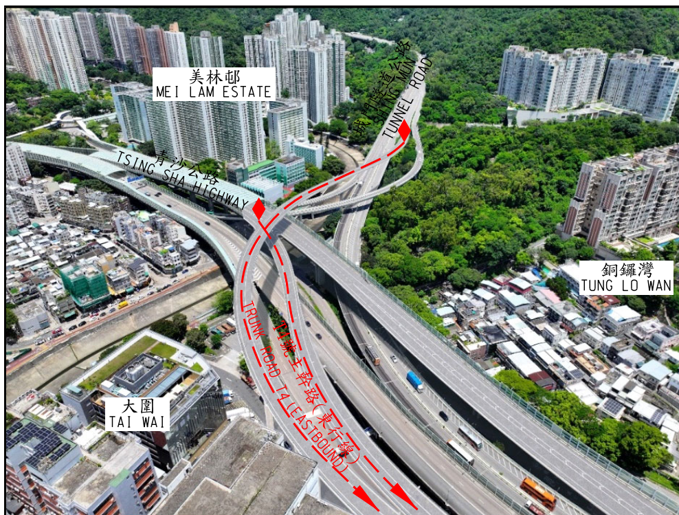
城門隧道公路/青沙公路匯入T4號主幹路(東行線)的接駁點 CONNECTION POINTS OF SHING MUN TUNNEL ROAD /TSING SHA HIGHWAY TO TRUNK ROAD T4 (EASTBOUND)
