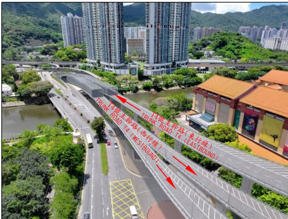
橫跨城門河道的高架行車道 VIADUCT ACROSS SHING MUN RIVER CHANNEL
