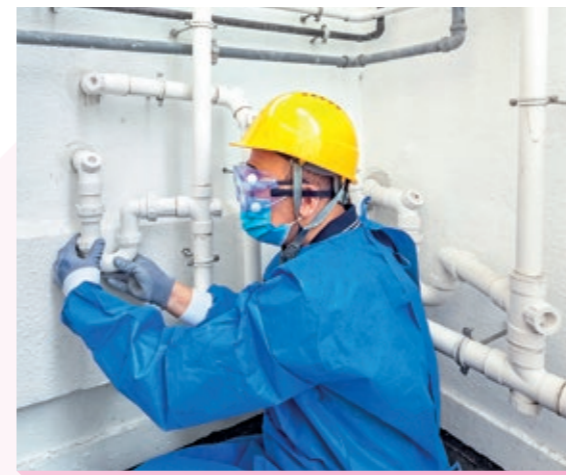
排水管改善計劃為居民檢查和改善排水系統 The DEP includes inspection and improvement works in estate drainage systems
