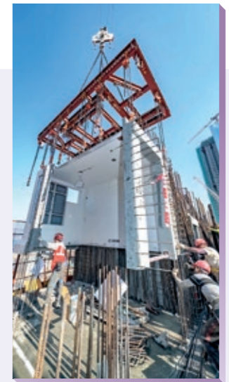
組裝合成建築法大幅減少組裝時間 Modular Integrated Construction significantly reduces installation time
