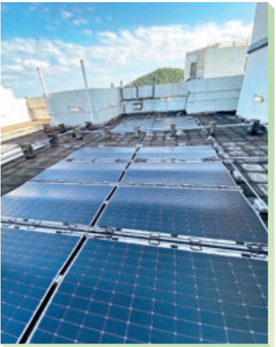
東區小西灣邨的柔性太陽能光伏發電系統 A flexible PV system at Siu Sai Wan Estate in Eastern District
